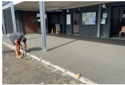
Concrete slab replacement 2026
