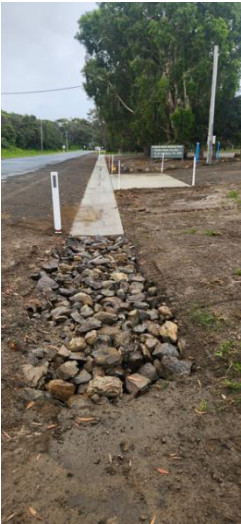
Street dish drain (2024)
