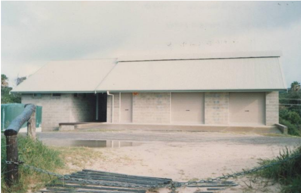
Stage 2 - toilet block
