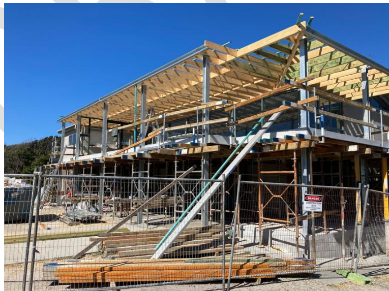
Stage 5 Deck & storage
