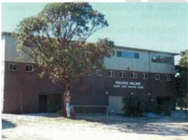
7 New extensions almost complete.
