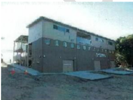
Recently constructed pathways
